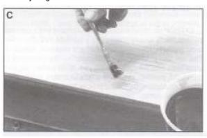
3. Cure the system and carefully remove excess sealant as in Picture D. Sanding will reopen the sealed surface and require a repetition of the sealing procedure.
