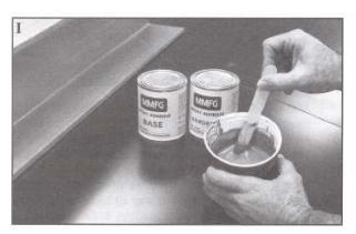
addition to the damaged section. The mechanical clamp supplied by the Fibrebolt will squeeze the epoxy into the damaged area. Do not permit the profiles to stand after applying the adhesive; proceed to the next stem immediately.
